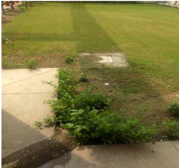
Fig.4. Underground rainwater tank.
