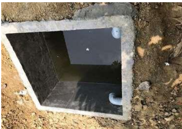
Figure 7: Rain Water Pit
