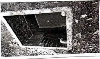
Rain water harvesting pit is installed to collect water instead of charging ground water.
