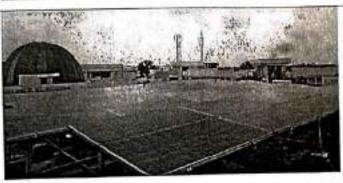
Cool roof may be provided with covering at roof level for exposed roof with broken china mosaic tiles. The Air conditioning energy for the top floor shall be reduced to the extent of 15 %
