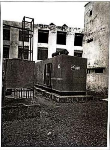
Stack of DG sets are not as per requirement of CPCB Guidelines. These are required to be taken above height of building and stack height should be as following formula
