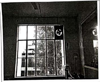
Exhaust hoods of Labs not provided for chemistry Lab fumes. The fume hood is required to be provided raised to level above building. The final exhaust should be raised above building for proper dispersion of fumes.
