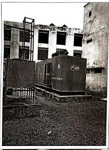
Stack of DG sets are not as per requirement of CPCB Guidelines.
