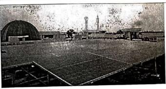
Cool roof may be provided with covering at roof level for exposed roof with broken china mosaic tiles. The Air conditioning energy for the top floor shall be reduced to the extent of 15 %
